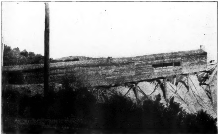
Detail of Housing for Waste Material Distribution
